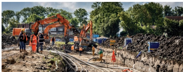
Figure 2: Direct Burial. Source: Europacable
