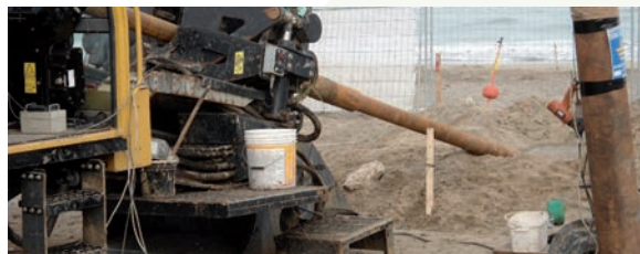
Figure 3: Horizontal directional drilling. Source: Terna
