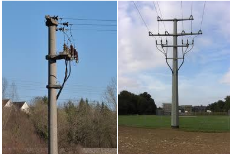
Examples for the transition from overhead line to cables
