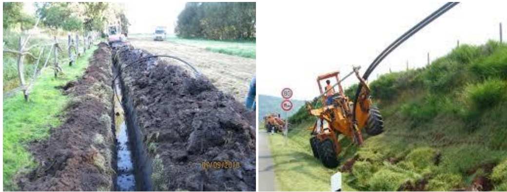
Examples for installation in open trench and by direct ploughing
