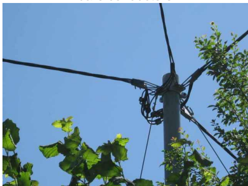
Example for a LV-ABC overhead line
