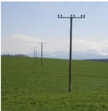
Example for a medium voltage overhead line with bare conductors
