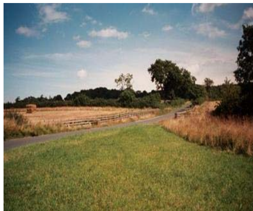
Figure 12 : cable route above ground
