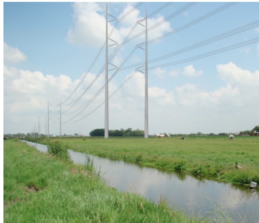
Image: 380 kV Wintrack pylons of the Randstad Project. Source: TenneT
