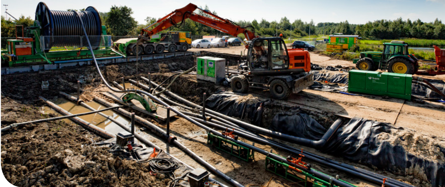
Image: 380 kV cable pulling in open trench with two systems. Source: TenneT
