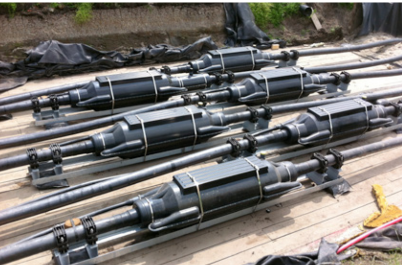
Image: The Joint Bay of the 380 kV double system after installation Source: nkt cables
