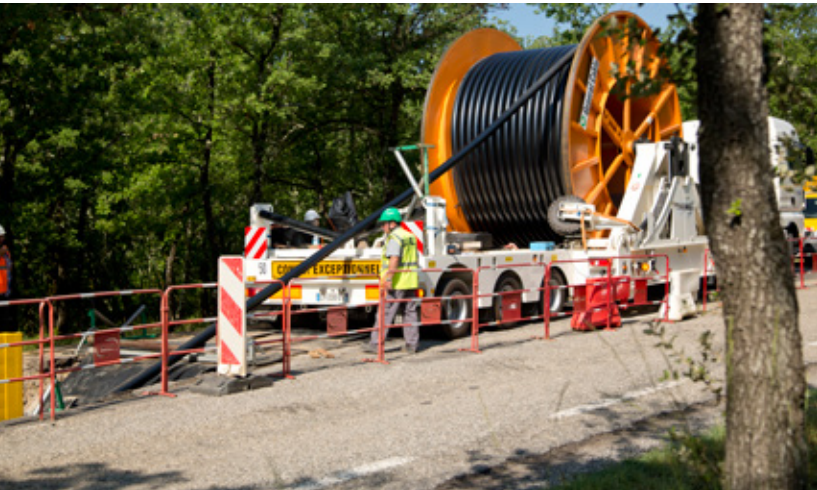
Image: On-site pulling operations of EHV cable. Source: General Cable
