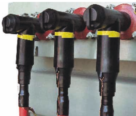
Figure 45 – Screened separable 'T' connectors (or 'elbows')
