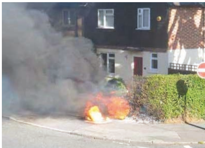
Figure 46 – Failure of a joint installed in a manhole under a walk-way
