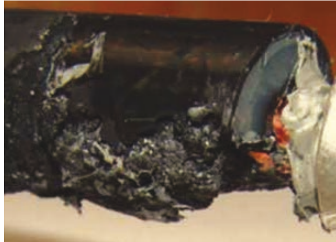
Figure 53 – Immediate failure due to insulation screen not being removed during installation
