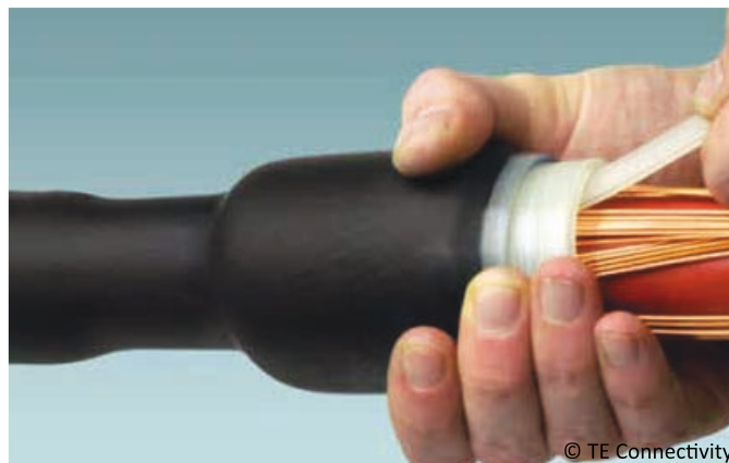
Figure 44 – Installation of a cold-shrink joint sleeve with spiral tape holdout
