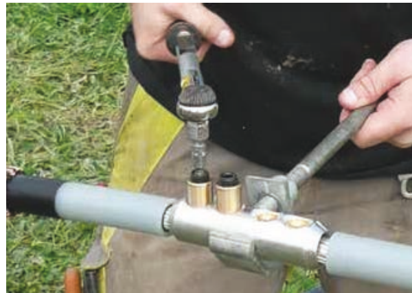
Figure 39 – Bolted connector with hexagonal socket screws
