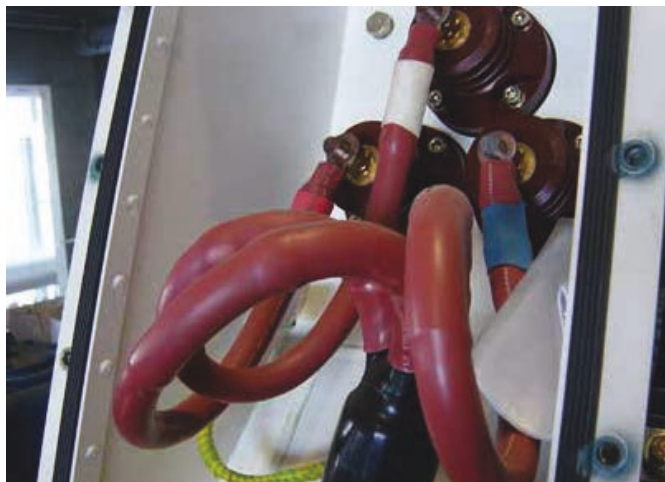
Figure 52 – Termination made without regard to dimensional instructions
