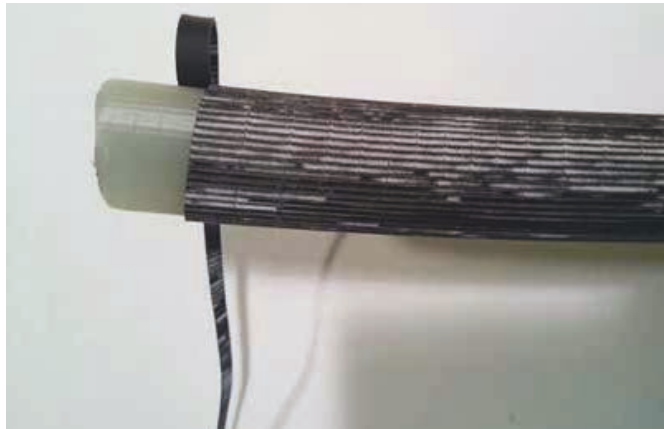
Figure 48 – Cuts into XLPE insulation caused by strippable screen scoring tool blade set too deep
