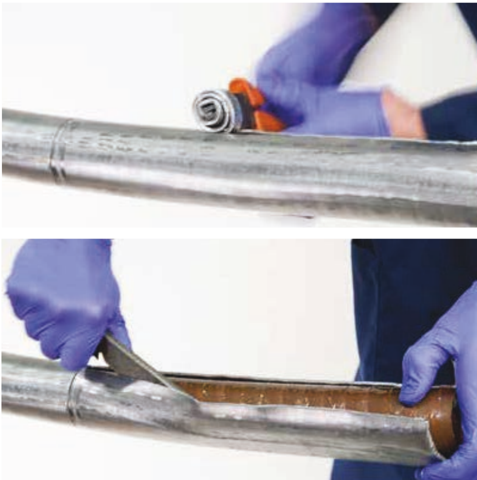
Figure 33 – A technique for removing lead sheaths
