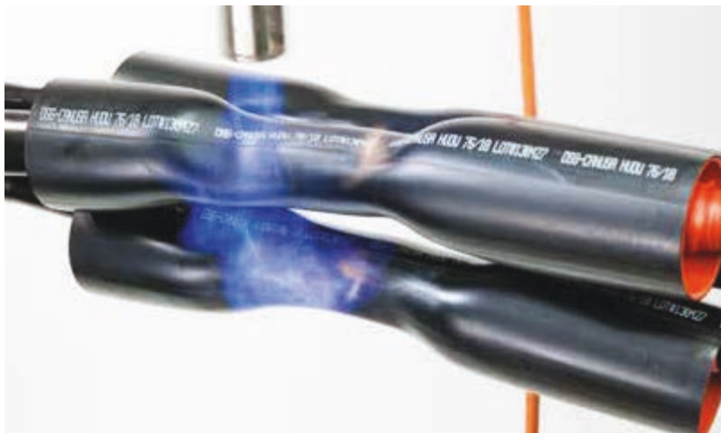
Figure 43 – Shrinking joint insulation/screening tubings
