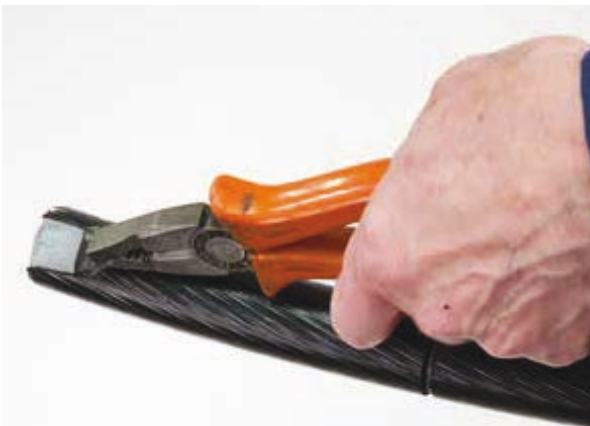
Figure 21 – Peeling strips of screen
